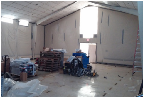
The old sanctuary, completely gutted for its makeover
