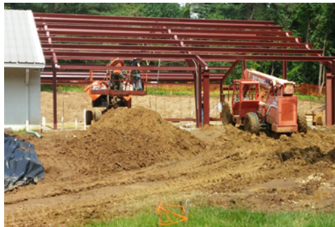
The steel skeleton erected for the new academic wing
