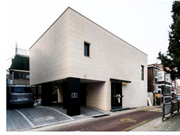
Outside of the new sanctuary and manse
