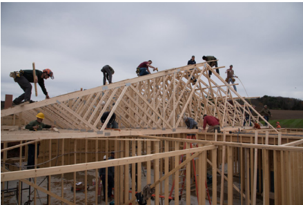
Volunteers working on the roof
