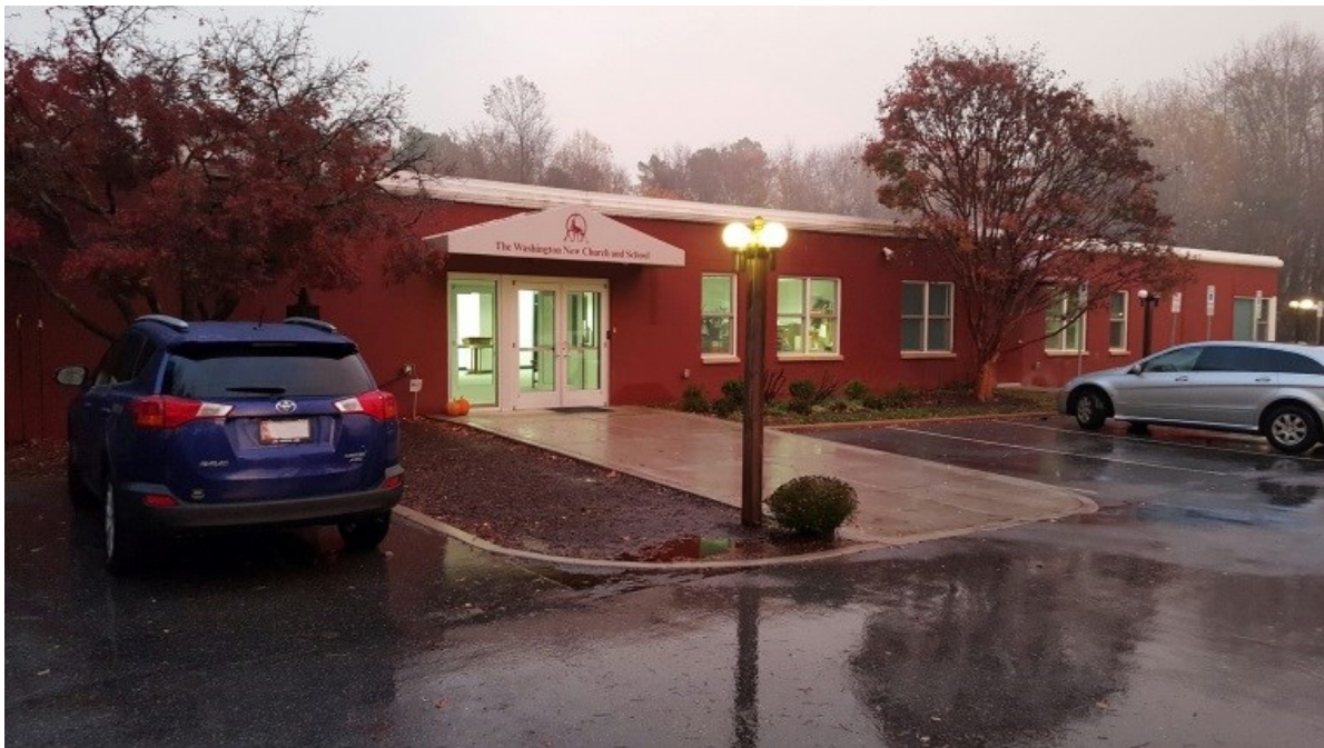
This photo shows the new outside entrance with its handicapped access ramp illustrating the fact that the entire building is now free of steps and “handicapped accessible.”
